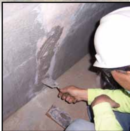
Treating crack with ChemLine® Caulk.
