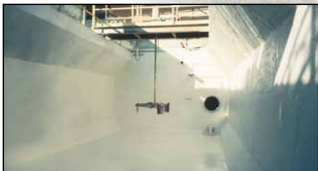
Finished ChemLine® Primer application over concrete surface.
