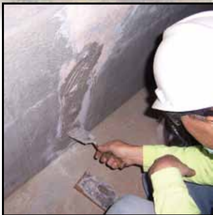
Treating crack with ChemLine® Putty.
