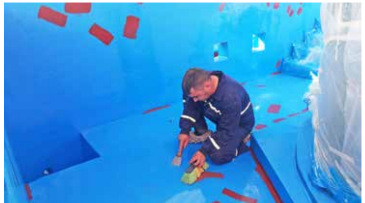
After the primer coat of ChemLINE® is checked, stripe coating of ChemLINE® base coat (red color) is applied where needed.
