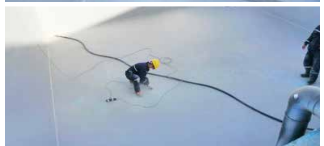
The concrete secondary containment areas are then lined with a ChemLINE® base coat (red color) and then followed with a ChemLINE® top coat (grey color) to finish out the protective lining application.
