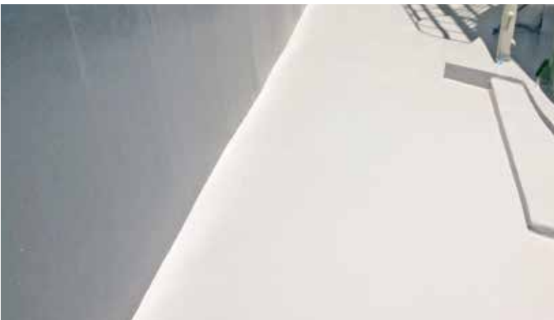
The concrete secondary containment areas are then lined with a ChemLINE® base coat (red color) and then followed with a ChemLINE® top coat (grey color) to finish out the protective lining application.
