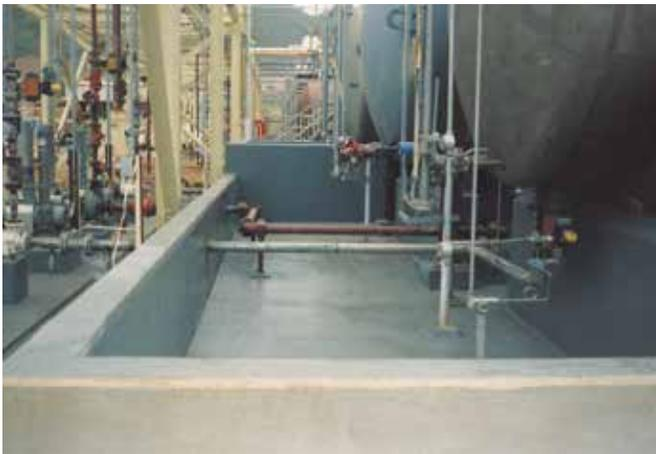
*ChemLine® coating for concrete protection.*
