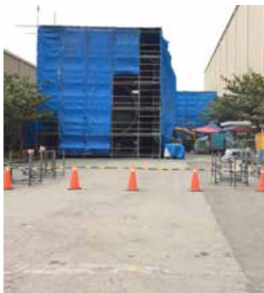
Setting up the tenting and staging for the blasting operation
