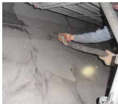
Grit-blasting to proper surface profile
