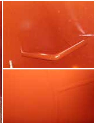
Applying the base coat of ChemLine® 784/32 (red colour)
