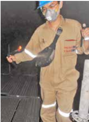
Inspection of blasting
