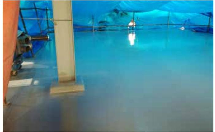
*Inside the covered staging area, heat curing furthers the protective cross-linking capability of ChemLINE®.*
