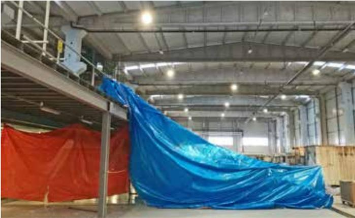
*After coating application, staging is set up in order to provide a high temperature heat cure to the coating.*
