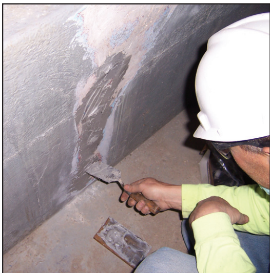
Treating crack with ChemLine ® Caulk.
