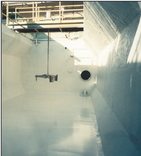
Finished ChemLine® Primer application over concrete surface.
