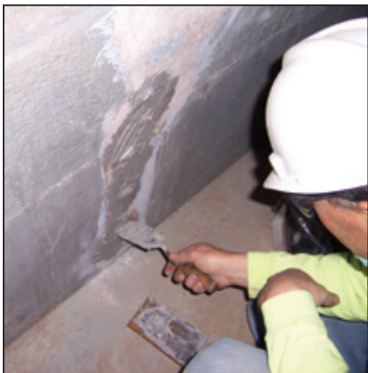
Treating crack with ChemLine® Caulk.
