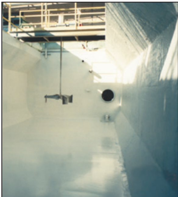
Finished ChemLine® Primer application over concrete surface.
