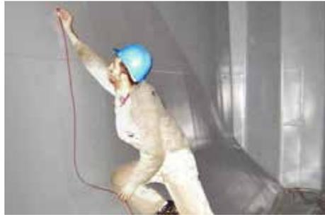
*Applying thermocouple to monitor temperature during heat curing of the cargo tank coating.*
