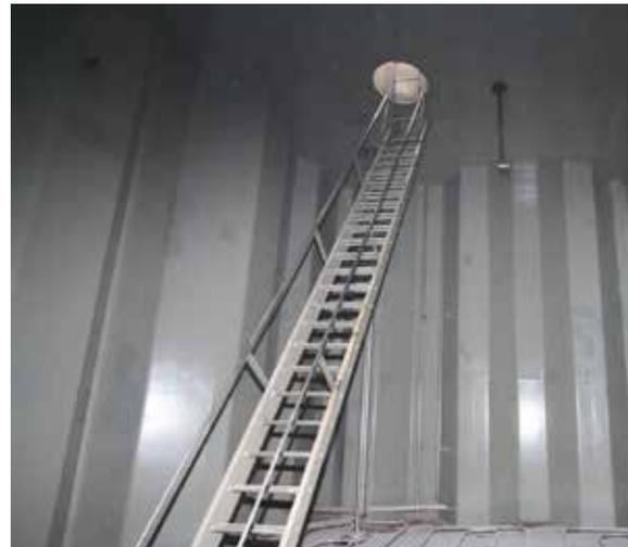
*This cargo tank from a chemical tanker, coated with MarineLine®, has successfully carried many loads of Methanol during its 5 years of service. This photo was taken during a recent on-board inspection of the coating. Only minor touch-up tank coating repairs were needed and the ship was quickly put back in service. The ship owner was very pleased with the ongoing performance of MarineLine®.*
