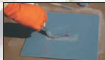
5. Applying MarineMend® to surface.
