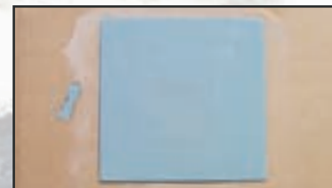
6. Finished and completed repair.
