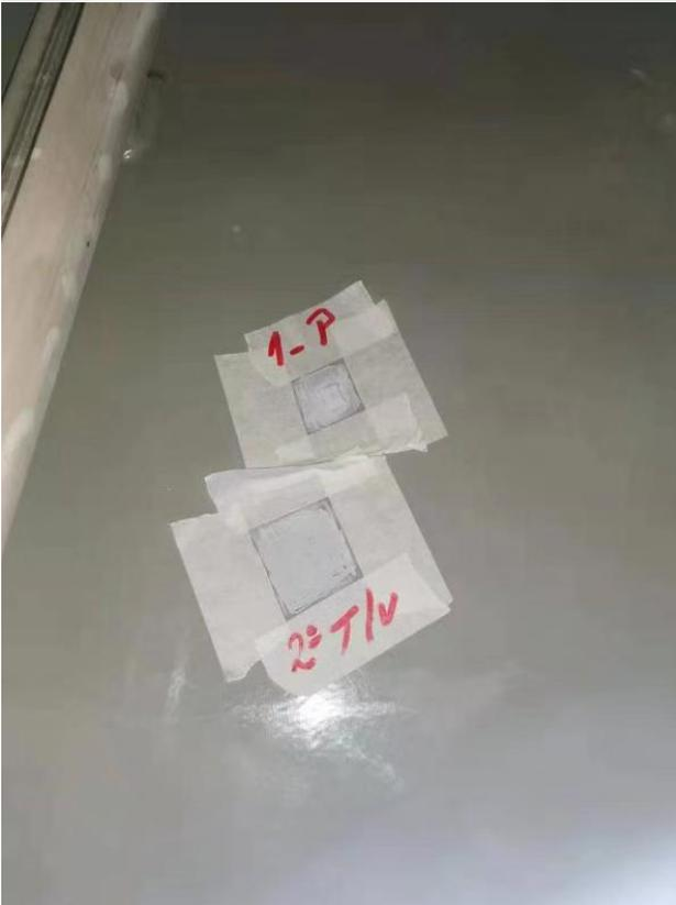
Touch-up with MarineMend repair kit (first coat Grey color). After the first touch-up is hard dry, which may be up to 24 hours depending on the temperature and air flow, sand smoothly by sandpaper before second touch-up.
